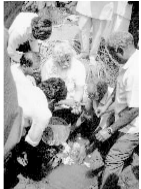
The shankusthapana (consecrating the foundation) of the new kitchen building in Adivarapupeta.
